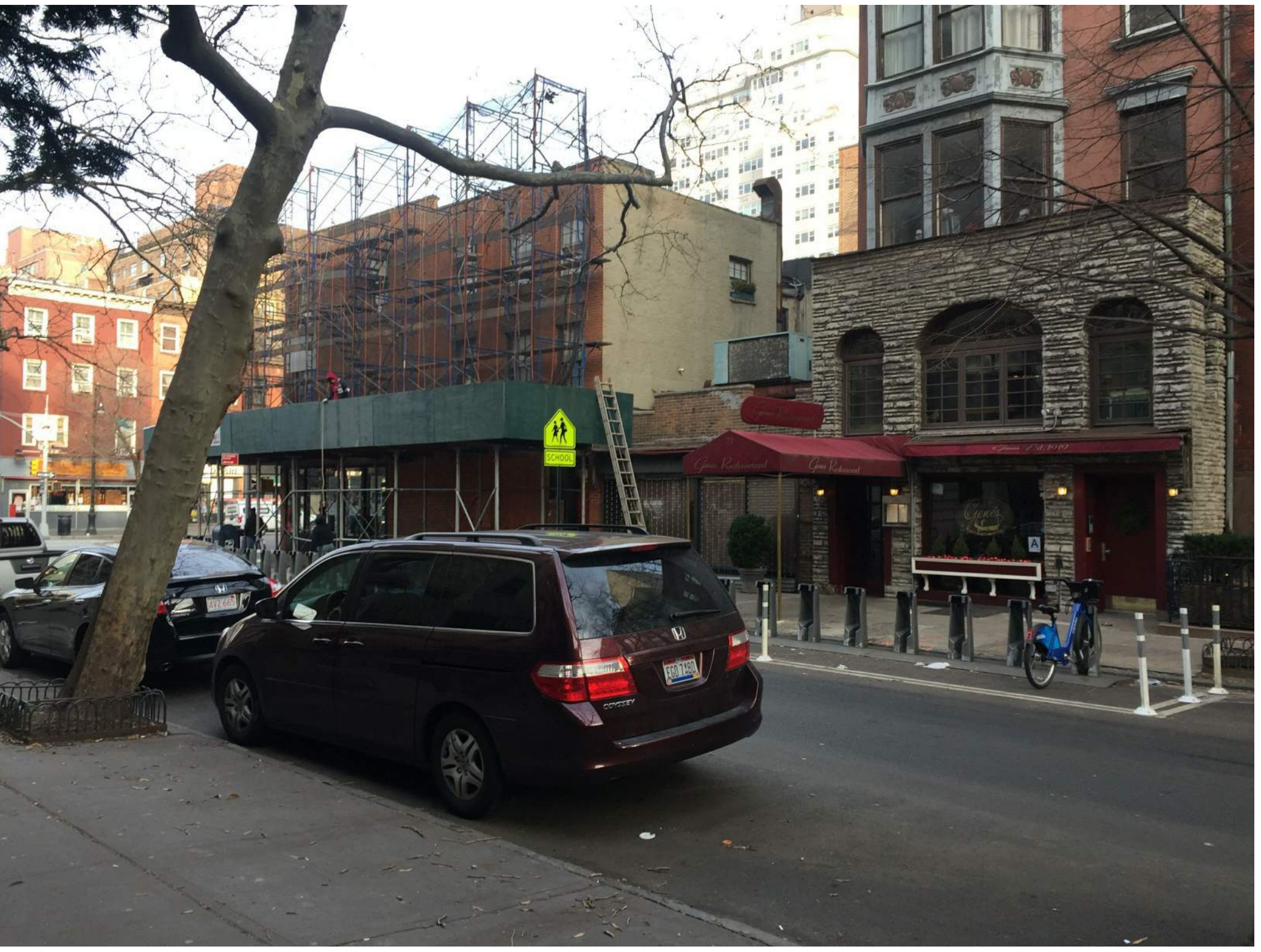
② Standing on corner of 6th Ave looking toward N.E. on 11th St.
