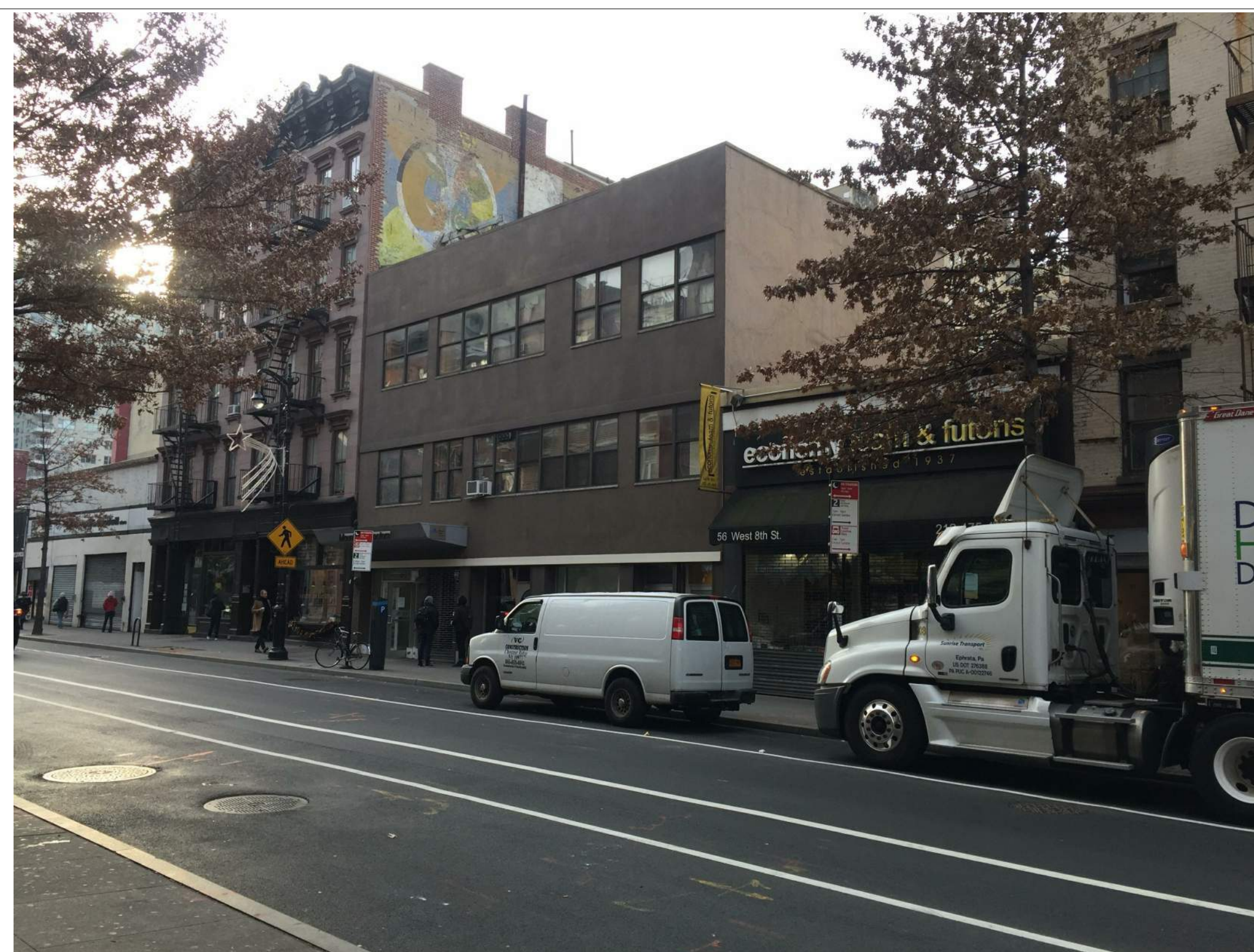
(F) Standing on corner of 6th Ave looking toward S.E. on 8th St.
